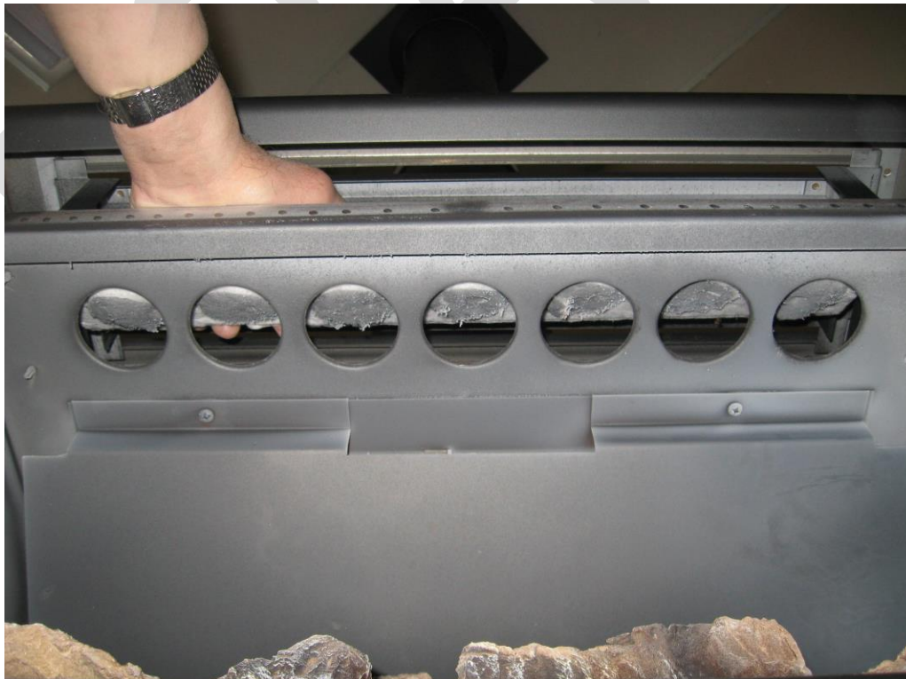
Pressure Relief Openings on Top of Firebox
